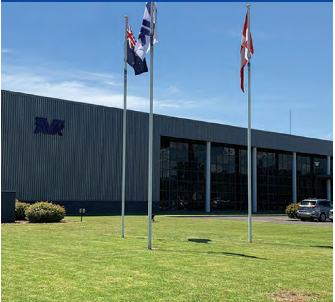
AVK Australia's Head Office | Wingfield, South Australia
