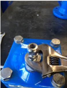
3. Hold air valve discharge fitting with appropriate spanner. This ensures that it will not turn and over tighten. (If this is not done and over tightening occurs this will distort the internal fitting and may jam the float which will not operate correctly).
