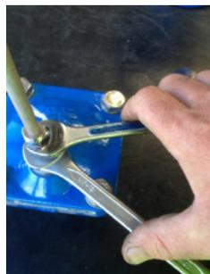
5. Insert stainless steel tube ensuring it bottoms out on male connector, use appropriate size spanner to tighten ferule nut while insuring the male connector body is held in position as not to turn.
