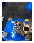
3. Hold air valve discharge fitting with appropriate spanner. This ensures that it will not turn and over tighten. (If this is not done and over tightening occurs this will distort the internal fitting and may jam the float which will not operate correctly).
