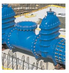
The standard axial adjustment of  $\pm$  60 mm offers a high level of flexibility in the installation and removal of flanged equipment for either maintenance or replacement. Larger adjustments can be accommodated if required.
