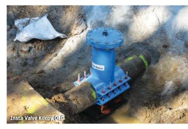
Insta-Valve<sup>®</sup> is not guaranteed to provide 100% shutdown. Insta-Valve<sup>®</sup> will provide a workable shutdown for pipeline maintenance, often achieving 100%.
