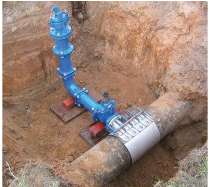
TUP Hydrant Installation at Casterto
